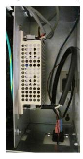
15. Secure the ground wires (GREEN with YELLOW stripe) from the mounting plate and AC Power Inlet Cable to one of the grounding lugs inside the mounting enclosure, as shown on the left.
