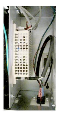
Figure 5: Fully Connected Power Supply, Front View
